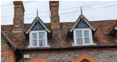
Gabled dormer with brick chimney
