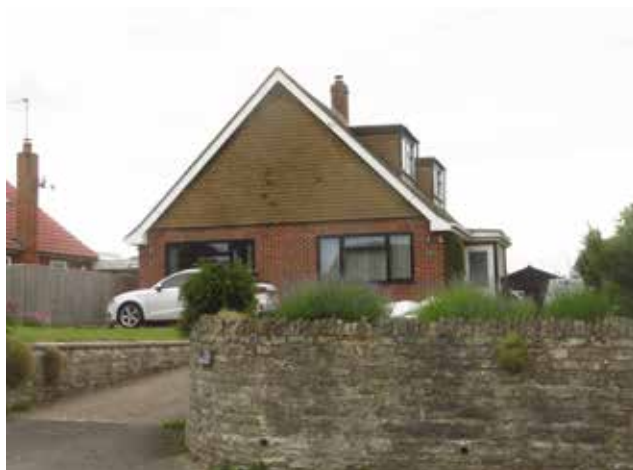
Figure 23: Local example of a renovated bungalow along Blewbury Road.
