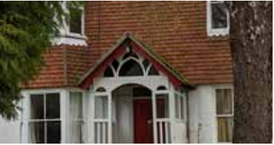
Gabled porch with wooden details
