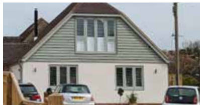
Half weatherboarding & half off-white render
