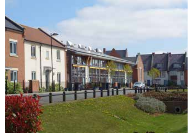
Figure 82: An example of a SuDS corridor - Upton Urban Extension, Northampton.
