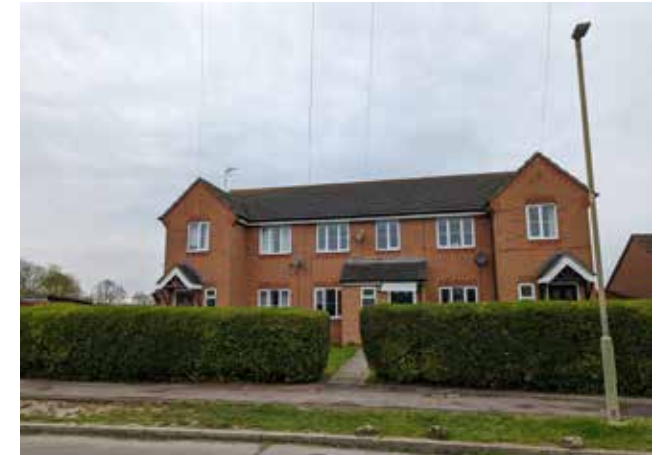
Figure 29: Example of thick hedges being used as boundary treatment within the character area.
