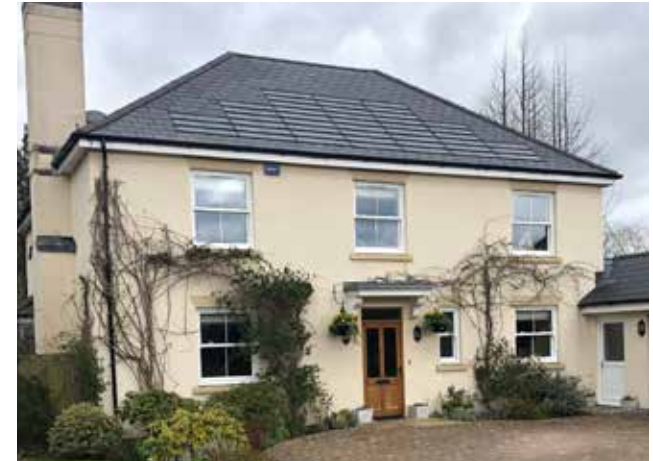
Figure 94: Use of shingle-like solar panels on a slate roof, with the design and colour of the solar panels matching those of the adjacent slate tiles.
