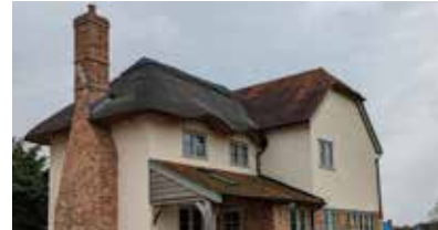
Thatched roof attached to a mansard roof and a brick chimney on a new home in East Hagbourne
