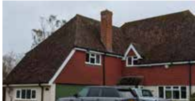
Half-hipped roof with clay tiles
