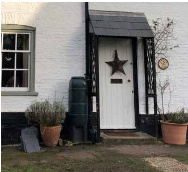
Figure 85: Examples of water butts used for rainwater harvesting in Reach, Cambridgeshire.
