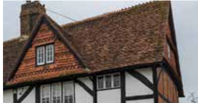
Cross-gabled roof with clay tiles and brick chimney
