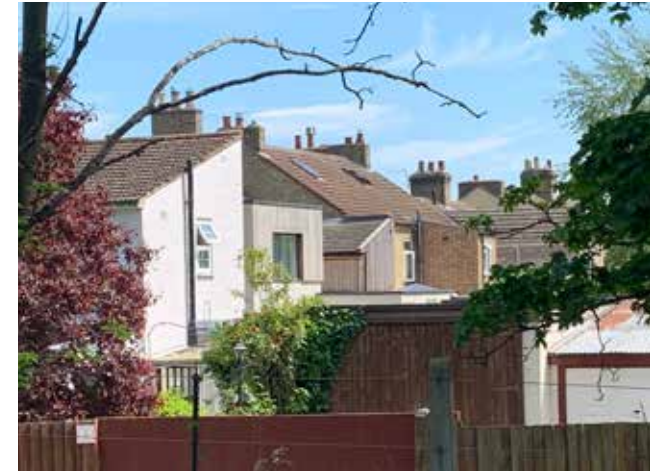
Figure 59: Positive example of a rear extension.
