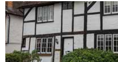
Timber frame with rendered brick
