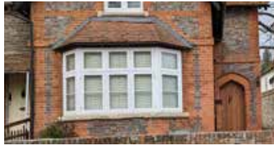
Bow window with hipped roof
