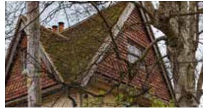
Tile hanging applied to decorative gable ends
