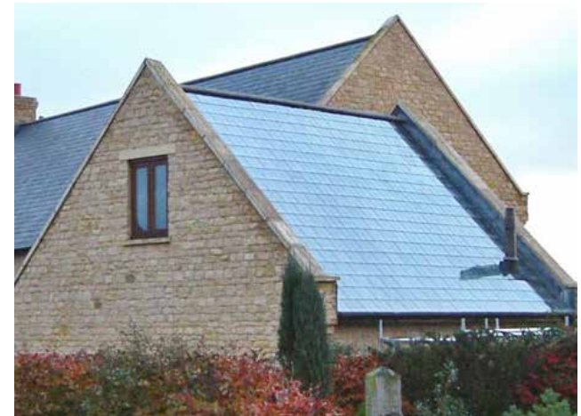
Figure 95: Positive example of implementing solar panels since the design stage.
