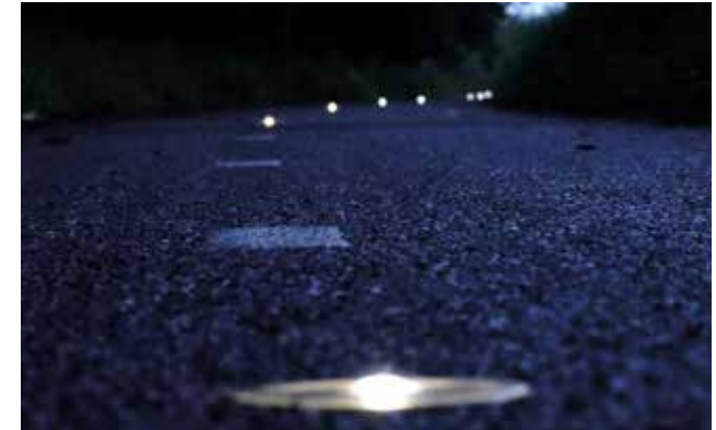
Figure 64: Example of a foot/cycle path which is lit by solar cat's-eye providing some light for pedestrian and cyclists without creating any disturbance to the nearby properties or unacceptable levels of light pollution.
