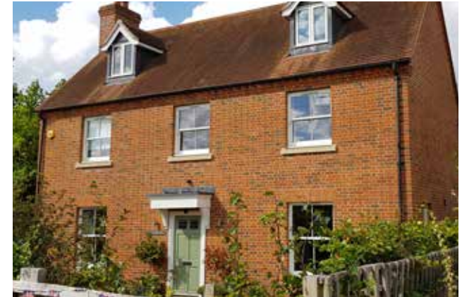
Figure 50: Local example of 2.5-storey building where the roofline is interrupted with a brick chimney and gabled dormers.
