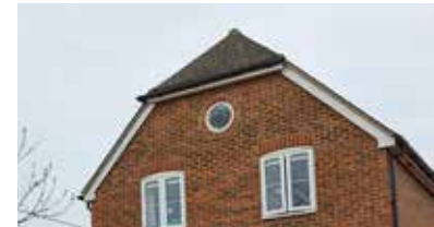
Dutch roof with clay tiles
