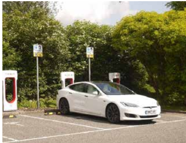
Figure 97: Example of electric vehicle charging points in a parking court.
