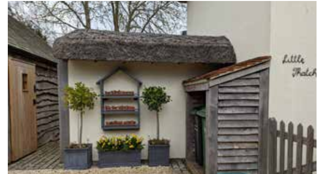
Figure 69: Local example where the bins are stored under the shed, whilst the side wall is decorated with flowers and plants to improve the environment. This arrangement combined with the particular permeable paving contributes to the rural feel of the village.
