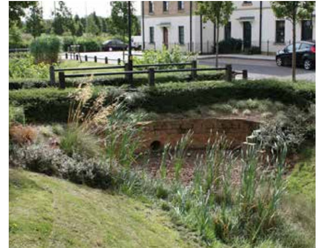
Figure 83: Example of swales check dam integrated with a crossing point, elsewhere in UK.
