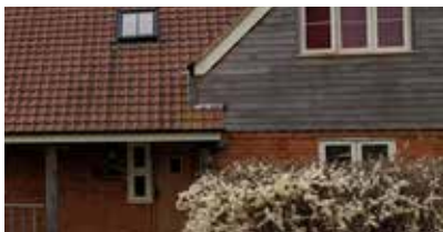
Half weatherboarding & red brick
