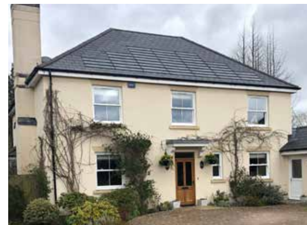
Figure 94: Use of shingle-like solar panels on a slate roof, with the design and colour of the solar panels matching those of the adjacent slate tiles.
