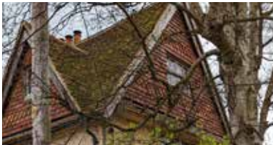
Tile hanging applied to decorative gable ends
