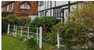
Stretch of painted metal railing
